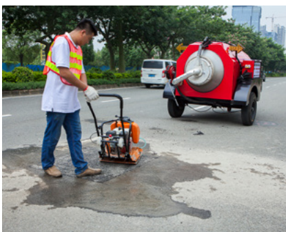
⑤ Compacted asphalt
