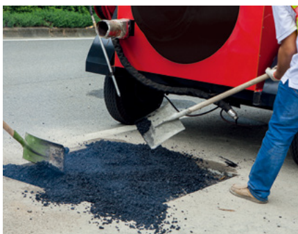
④ Discharge and pave
