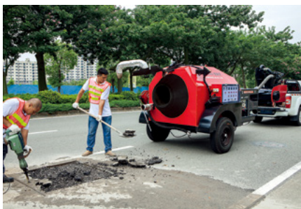
① Crush the damaged asphalt pavement
