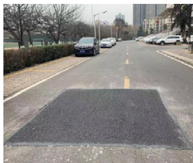
⑥ Patching complete
