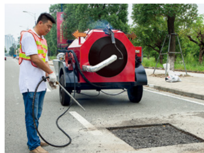
③ Set temperature for heating and regeneration
