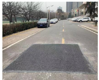
⑥ Patching complete
