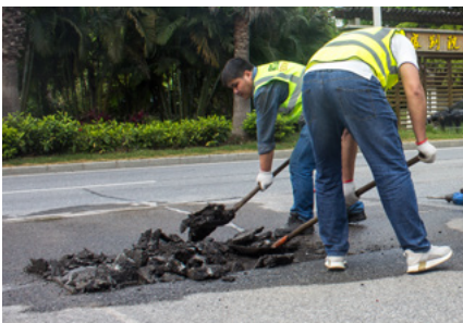
① Crush the damaged asphalt pavement
