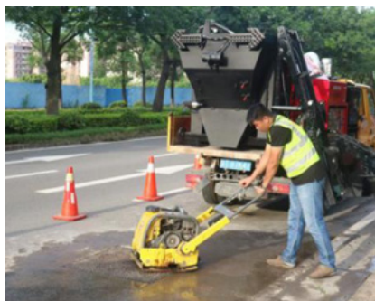
⑤ Compacted asphalt
