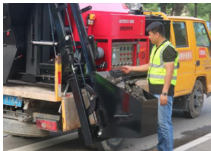
② Recycled the old material from hopper to roller heating box
