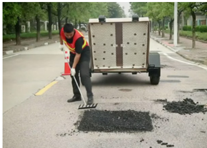
② Raking and adding new asphalt
