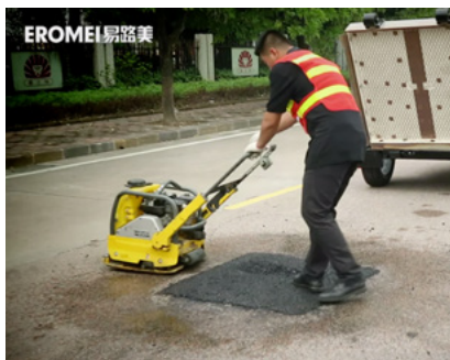
⑤ Compacted asphalt
