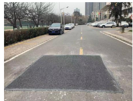
⑥ Patching complete
