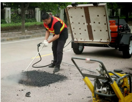
④ Spray emulsified asphalt
