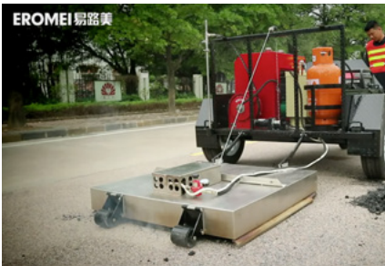
① Heating damaged asphalt pavement
